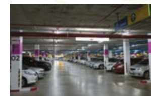
Underground car parks
